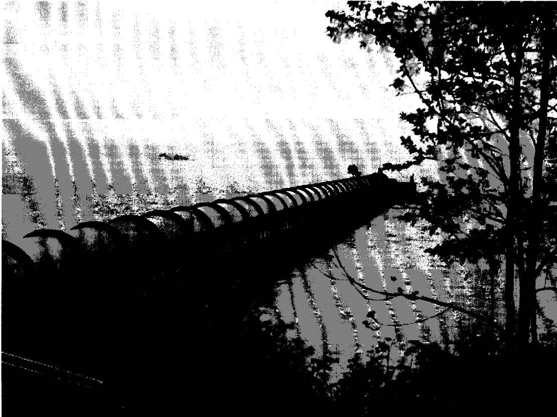
Figure 2- AES Greenidge Unit 4 Intake
